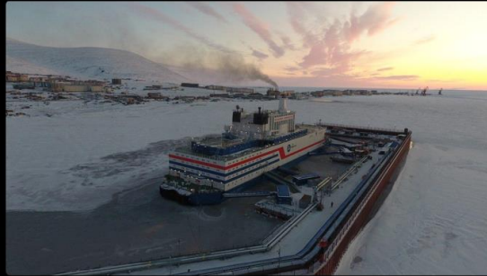
The world's first floating nuclear power plant Akademik Lomonosov
