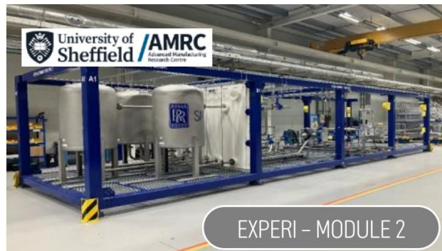
MEP Assembly of Complex Module
