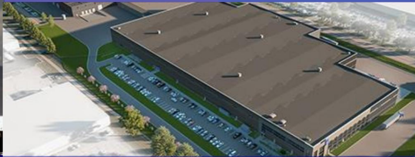
Data Center Backup Power
