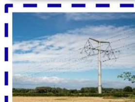
Grid Electrical Power
