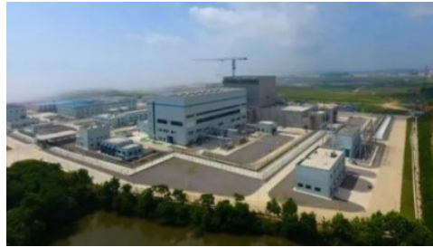
HTR-PM, China 2x110 MWe HTGR Under Commissioning
