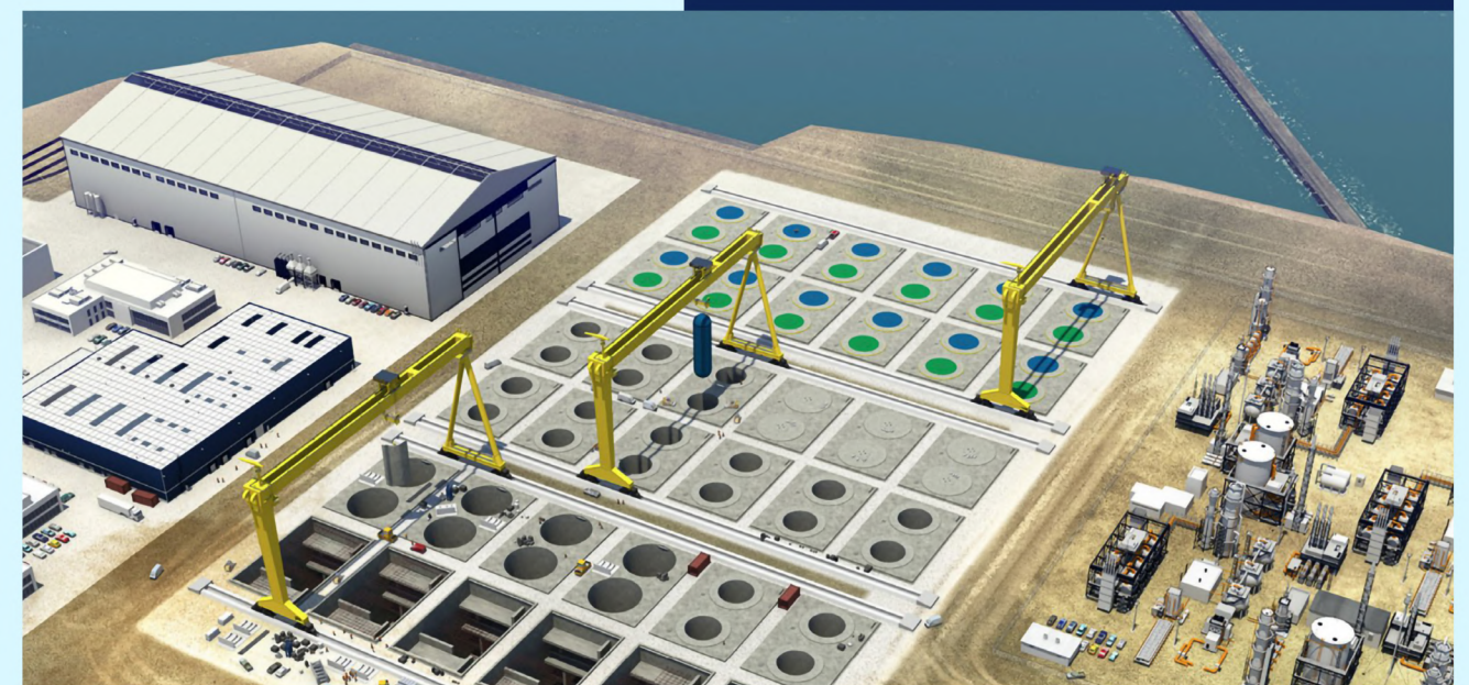
Figure 2: A Gigafactory making standardized reactor units at scale, which are used to populate the local hydrogen or e-fuels manufacturing plant operating at tens of gigawatts scale.
